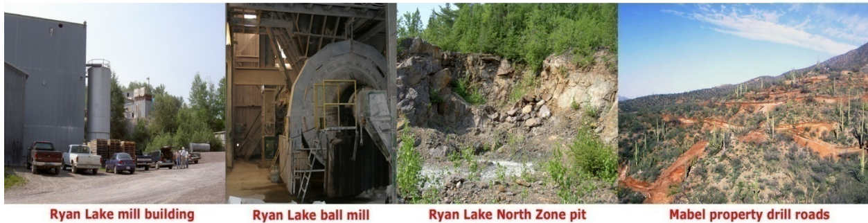
Ryan Lake mill building
