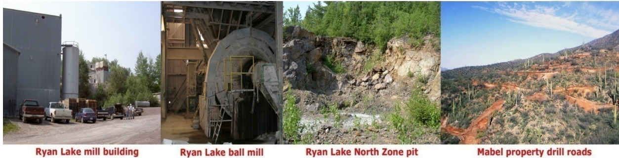
Ryan Lake mill building
