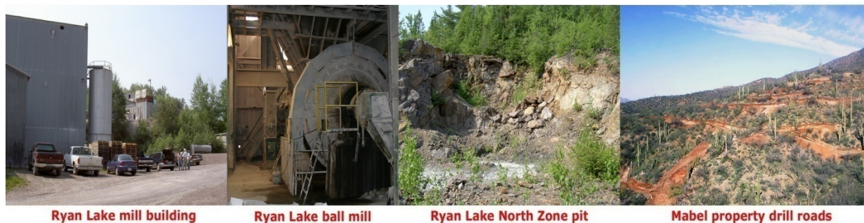
Ryan Lake mill building
